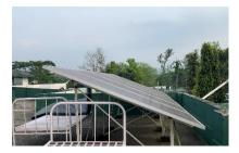
Solar energy is used as a backup, whenever there are power cuts. The solar power systems installed in the covid care centre and isolation ward have capacities of 3.96kW (12 solar panels) and 2.97kW (9 solar panels) respectively. In the case of unavailability of sun, the battery provides a backup of up to two days. The staff at the hospital has been trained for the maintenance of solar panels.
